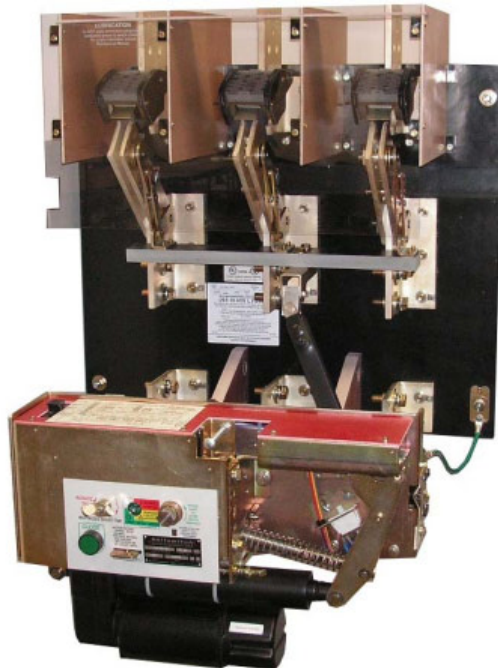
Figure 8 Sample Electrical Operator / Switch Assembly
