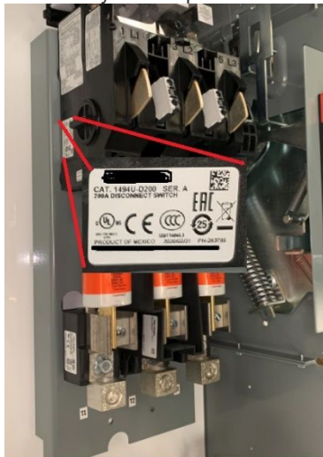
Fig. 2 Disconnect Switch with Certification Label
