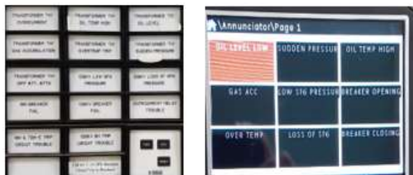
Fig.4 - Conventional and Digital Annunciator Panel
