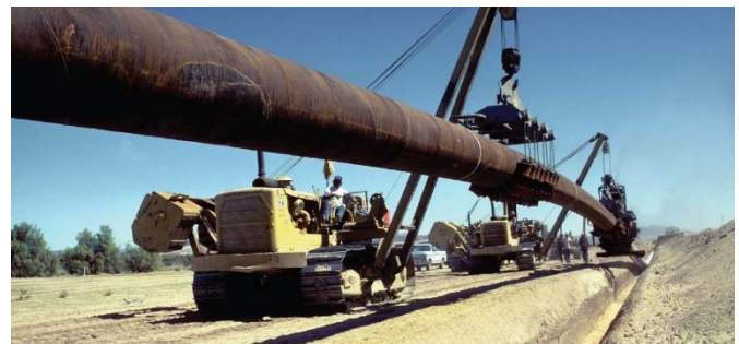
Fig. 1 Mangala Development Pipeline under construction
