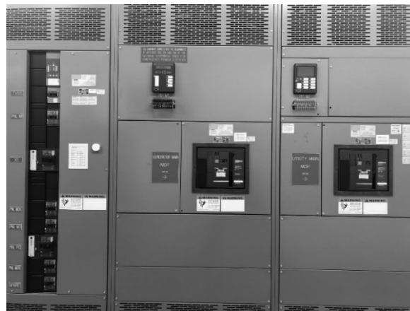
Fig. 1 Typical Service Entrance With Multiple Sources
