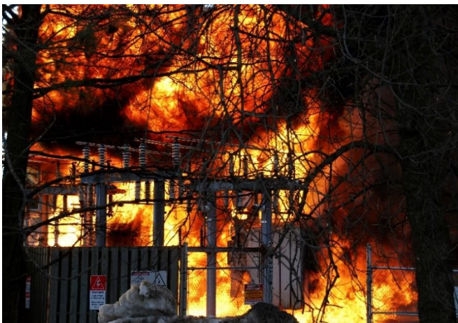
Fig. 1: Mineral Oil Substation Transformer Fire (Photo credit: Shutterstock)
