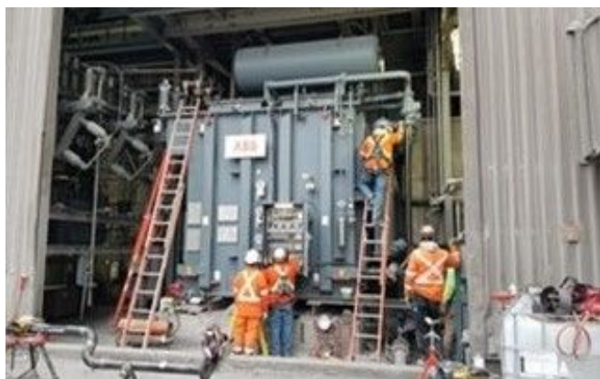
Fig. 4: A 47.8 MVA electrical arc transformer being retrofilled with synthetic ester liquid (Photo credit: Charter Steel, Saukville, WI)
