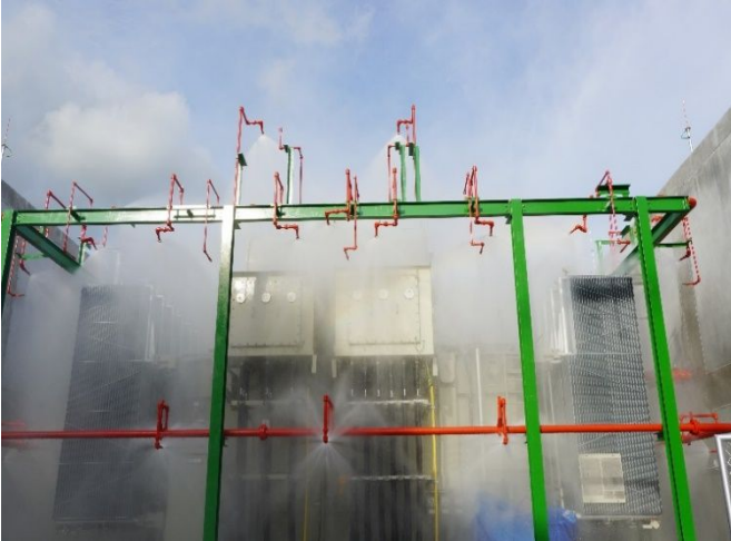
Fig. 2: Water Spray Transformer Fire Suppression System (Photo credit: Shutterstock)
