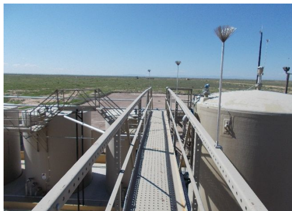
Fig. 1 CTS Devices Installed
