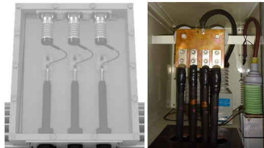
Fig. 4 Motor cable box – left; right; single phase with HVCC disconnected
