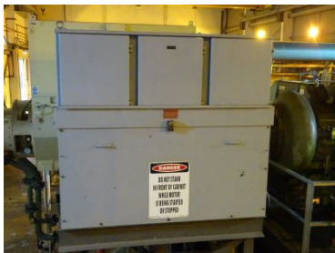
Fig. 3 9000HP, 4-pole, 6.6kV induction motor cable box
