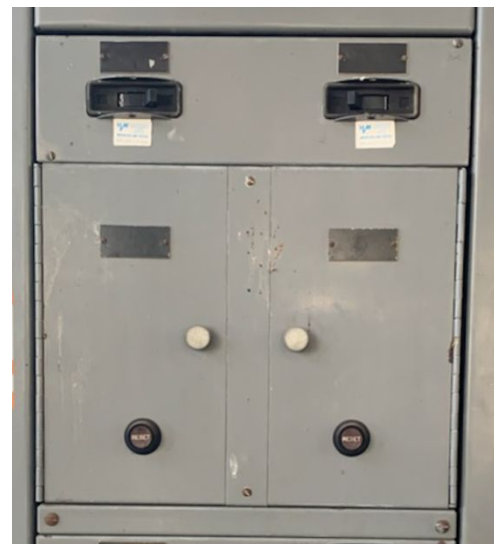
Fig. 1 480VAC MCC Bucket with Unreadable Nameplates
