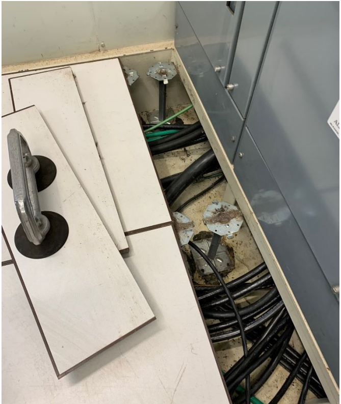
Fig. 5 Site 2: 480VAC and 129VDC MCC Sub-Floor
