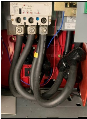
Fig. 2 Cable Spliced in Breaker Enclosure
