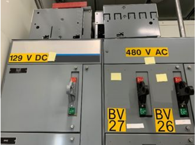
Fig. 4 Site 2: MCC with 480VAC and 129VDC Sections
