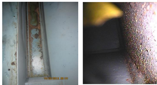
Fig 1 Presence of debris observed With evidence of insulation degradation, the key questions to ponder were:
