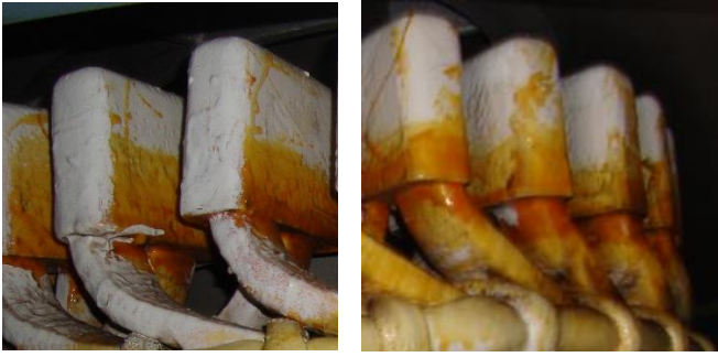
Fig 5 Resin exuded from insulation end caps
