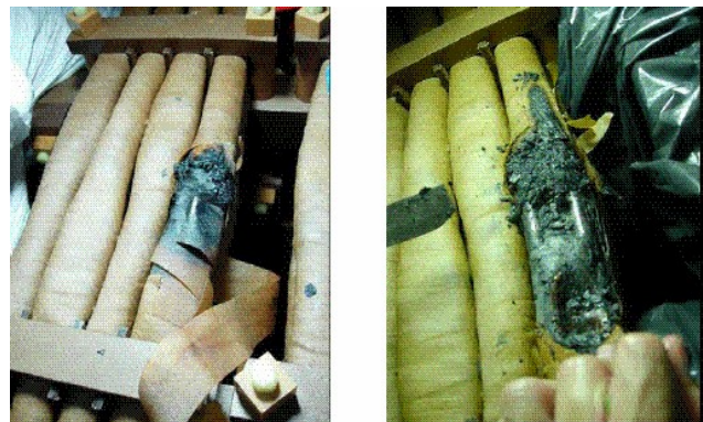
Fig. 13 Cable Nearly Burned Through
