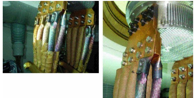
Fig. 12 Discoloration of LV Bushing Terminations
