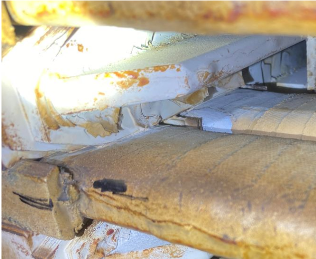
Fig. 4 Surface Partial Discharge Activity
