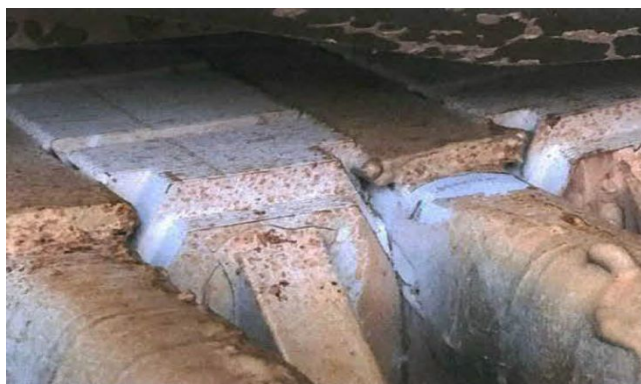
Fig. 17 Stator Winding at Slot Exit Locations (continued)
