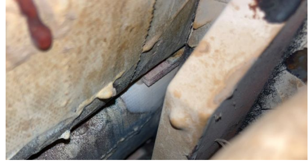
Fig. 20 Loss of Conducting Armor at Slot Exit Locations
