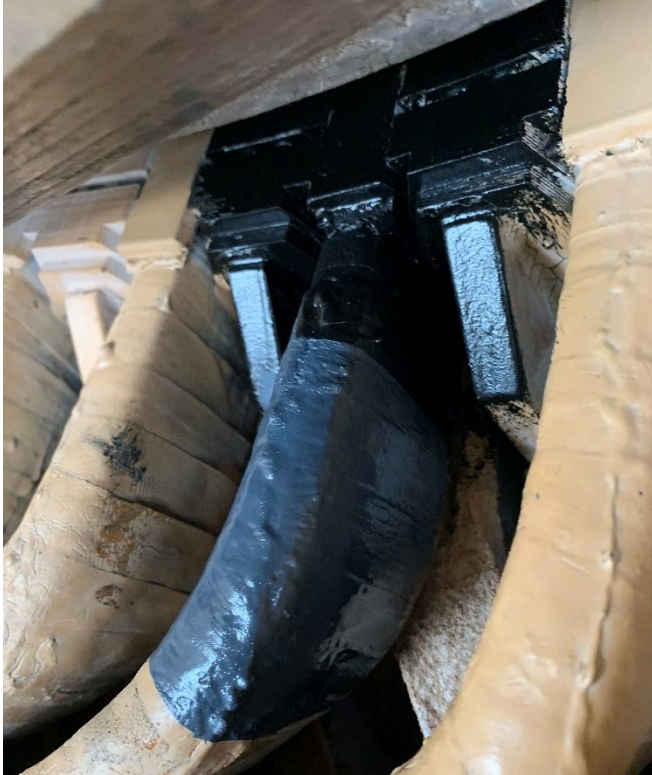
Fig. 26 Restoration of Corona Suppression System
