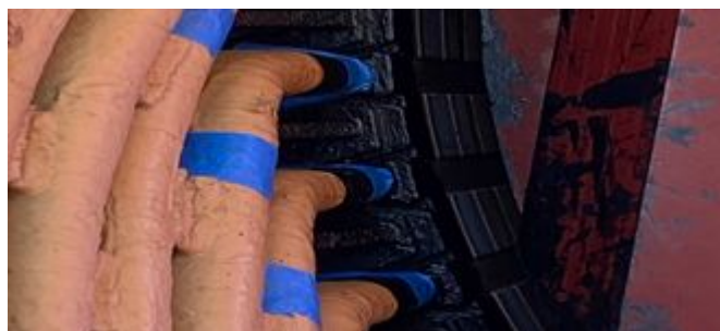
Fig. 11 Painters Tape Applied for Gradient Paint
