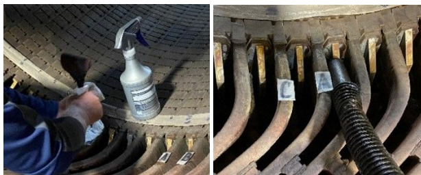
Fig. 8 Removing Excess Debris
