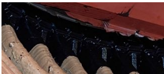
Fig. 10 Semi-con Paint Application
