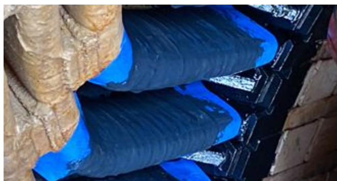
Fig. 12 Gradient Paint Layer Applied
