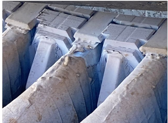
Fig. 25 Line-end Coil Showing Loss of Conducting Armor
