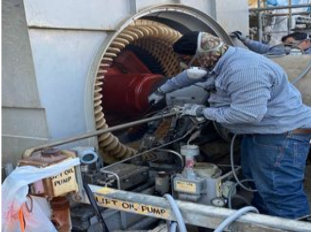
Fig. 13 Application of Two-part Epoxy
