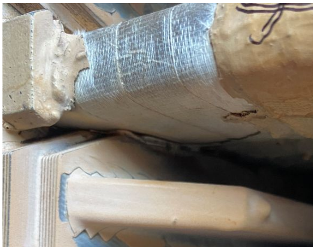
Fig. 5 Degradation to Conducting Armor at Slot Exit
