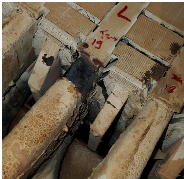
Fig. 17 Stator Winding at Slot Exit Locations
