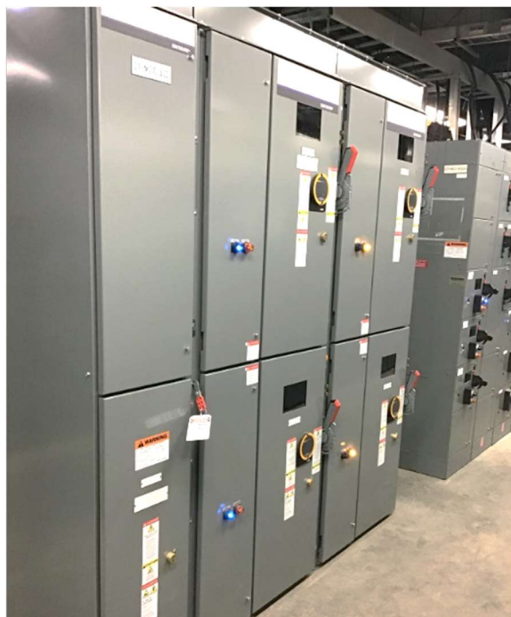
Fig. 5 New 4160V ASD Motor Control Center
