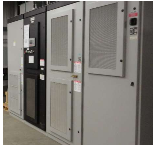
Fig. 4 1500 HP 4160 V Adjustable Speed Drive
