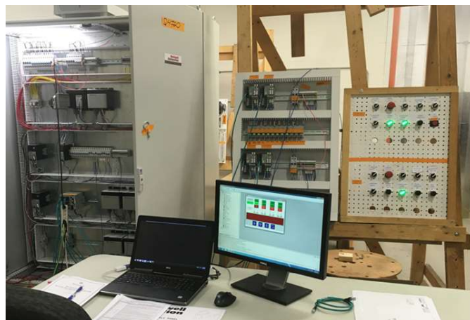
Fig. 6 Factory Acceptance Test of PLC Hardware and Program
